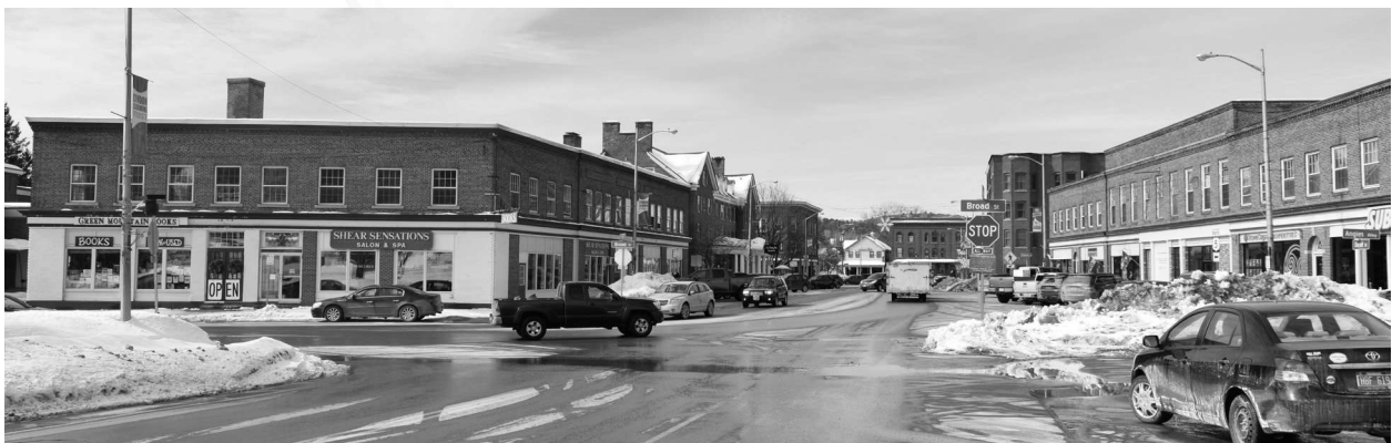
Intersection at Depot and Broad Streets. This view shows that the commercial blocks in town are mostly two-stories, with some taller exceptions. The streets are wide. Wires are underground. There is very little vegetation in the village core. This intersection is not pedestrian friendly.
